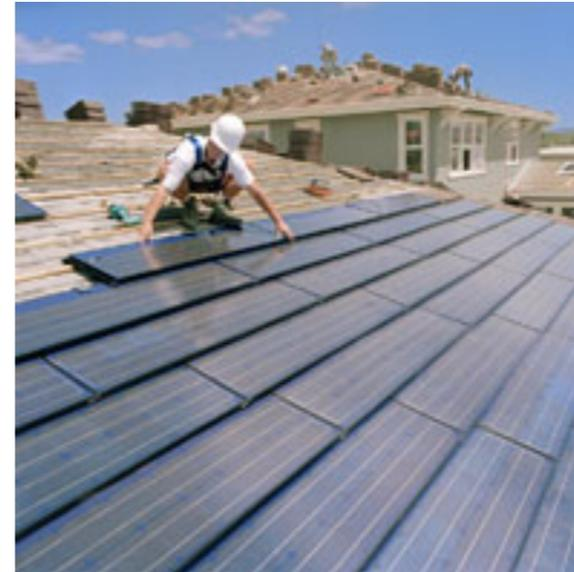
Aha!!—The Solar panel must take on the function of the roof tile
